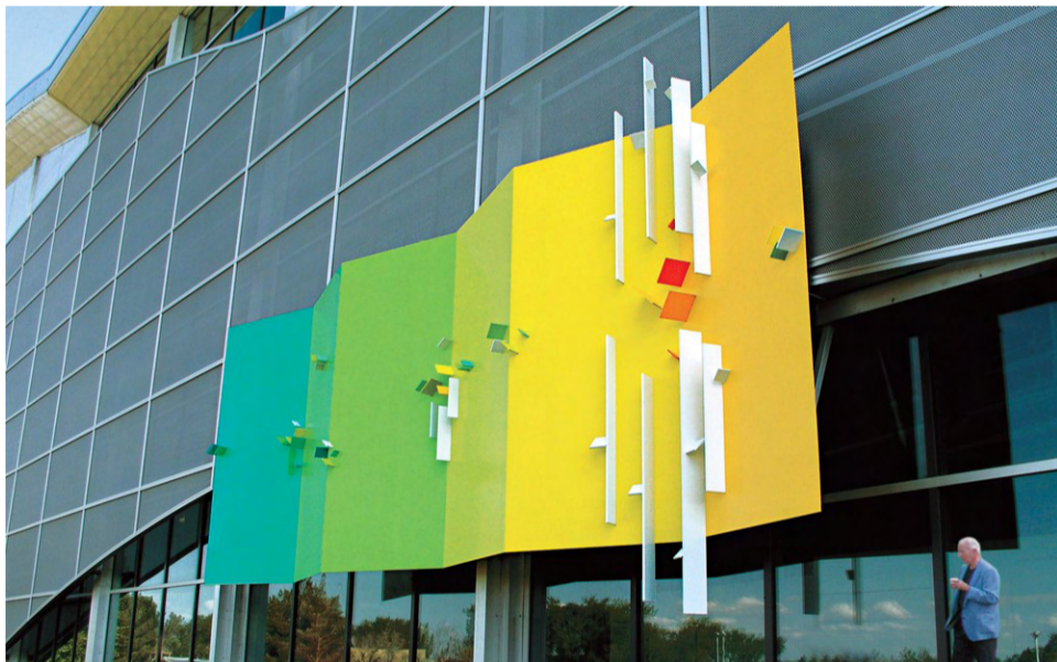
Installation view of Untitled Hexaplane Structurist Relief , 2004, by Eli Bornstein on the Canadian Light Source Building, University of Saskatchewan, Saskatoon, date unknown, photographer unknown.
